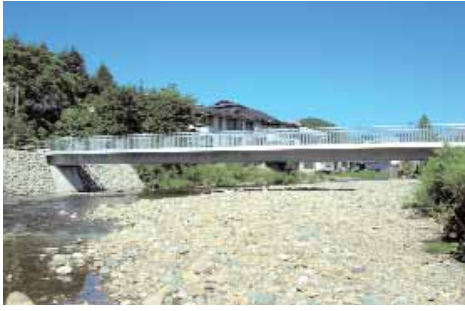
The footbridge at Yokemuri consists of a single span, 35.30 m long. The box cross-section has a constant height of 0.95 m and a total width of 3.50. The durability of Ductal® enables it to withstand the region's extreme climates.
