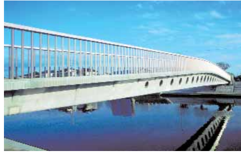
The Sakata Mirai footbridge in Japan: no passive reinforcement for this footbridge with a span of 50 m, a width of 2.4 m and a deck 50 mm thick.
