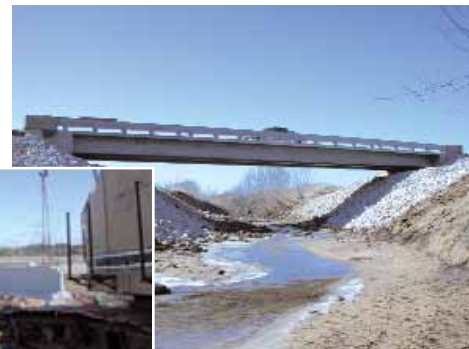
The test bridge in Wapello County Iowa: 3 girders with a span of 33 m: The simplicity of installation considerably reduces costs.
