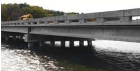
Cat Point Creek Bridge Virginia (United States)
