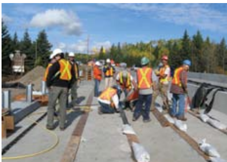
Hawk Lake Bridge Ontario (Canada)
