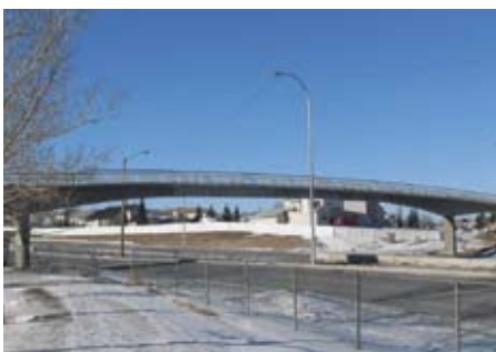
Country Hills Pedestrian Overpass Alberta (Canada)
