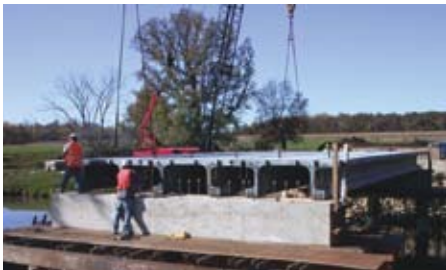
Jakway Park Bridge Iowa (United States)
