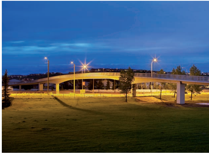
Ductal® Girder: Sanderling Drive Pedestrian Overpass, Alberta, Canada
