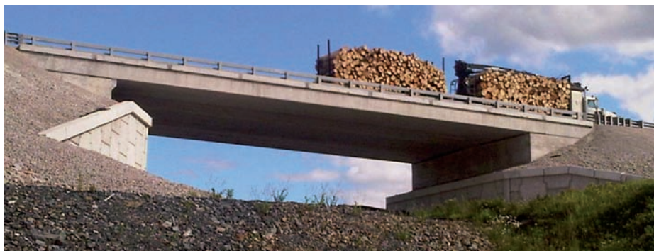
Ductal® Joint Fill: Hawk Lake Bridge, Ontario, Canada; PCA Concrete Bridge Award, 2010
