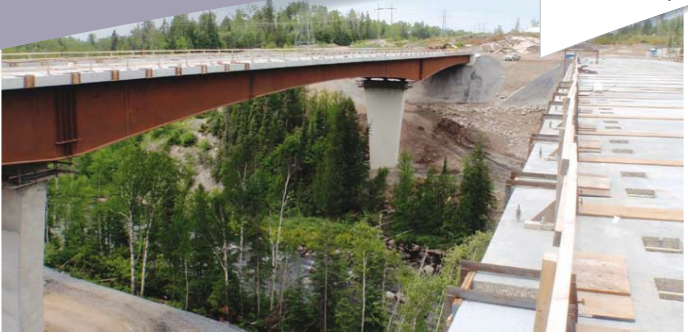
The Mackenzie River twin bridges near Thunder Bay, Canada: the largest field-cast Ductal® project in North America.
