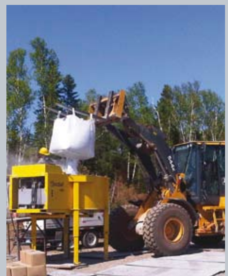
Mixing Ductal® on-site
