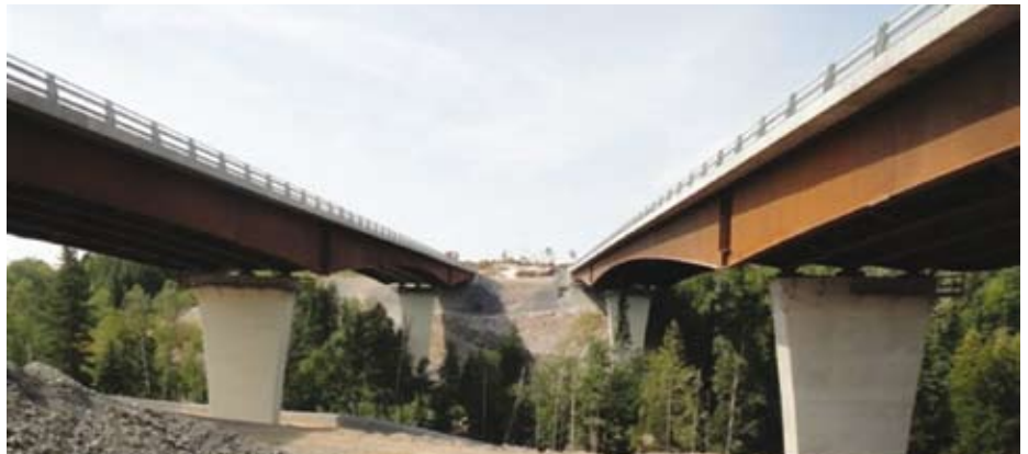
Mackenzie River Twin Bridges
