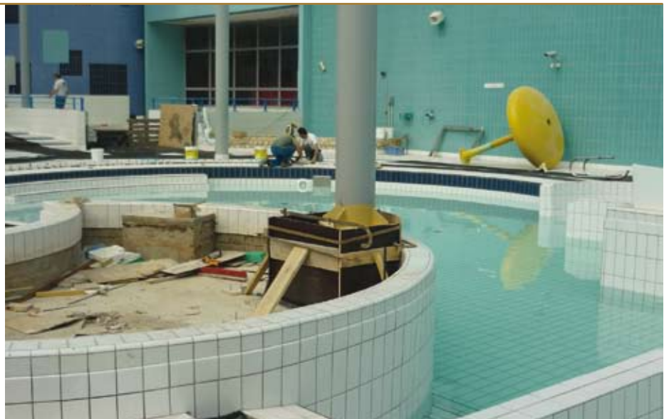
A renovated pillar base in the swimming complex
