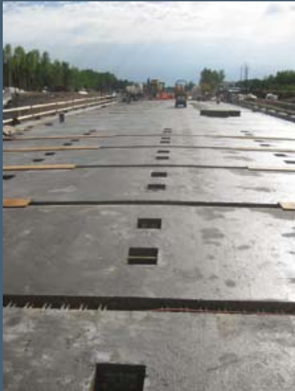
Precast bridge deck ready for joint fill
