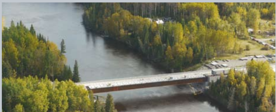
Chukuni River Bridge: the longest single span bridge in Canada
