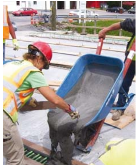
Placement of UHPC into the longitudinal connection between deck bulb-tee girders
